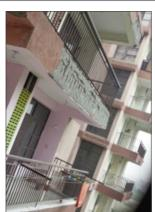
lying vacant. Due to the poor construction of the society. the plaster is falling all over. In all the constructions done by IRWO before today all in other society irwo use stone outside of the wall which gave a different identity to the construction of the houses of IRWO.
